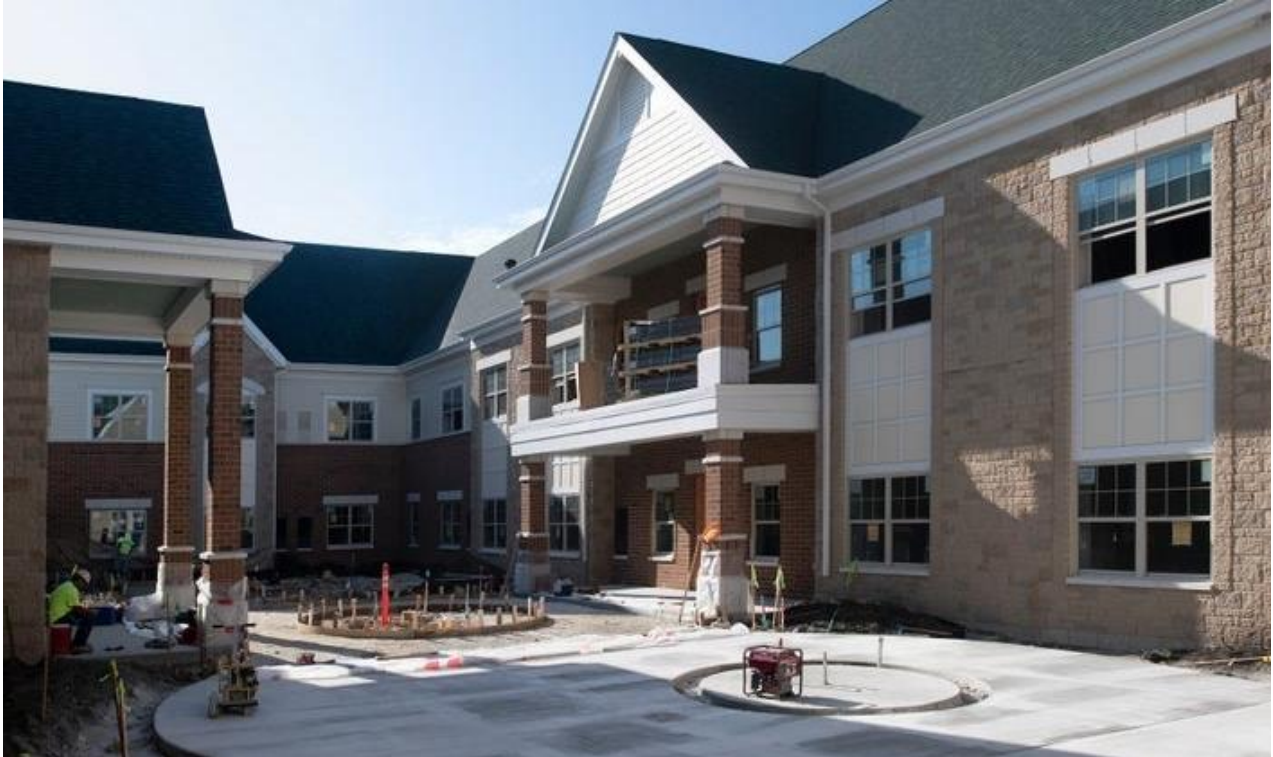
Smith Crossing in Orland Park will open its new short-term stay rehab wing early in 2020. (Smith Crossing)
